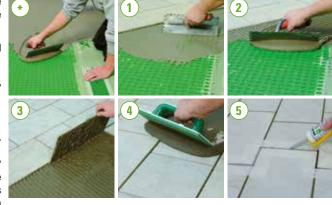
atmospheric agents and direct wear. Clean the surface thoroughly before applying the finish: removing dust, any condensation, residue from previous operations, and apply a layer of adhesive to fill the circular cavities, then cover the whole of the surface with an even layer of adhesive approximately 1-2 mm thick.
