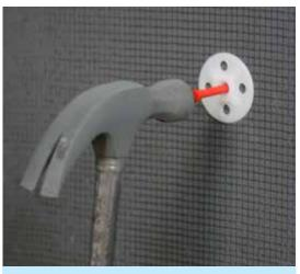
Once the adhesive has dried drill the holes out. Place the white dowel in through into the wall and then hammer in the pin.
