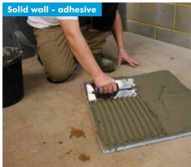
1 Use a 6/8mm trowel to comb adhesive over the who surface of the Marmox Multiboard. For uneven walls increase to a 20mm trowel.
