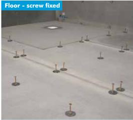
For screw fixing use a screw and Marmox washer at every 300mm.
