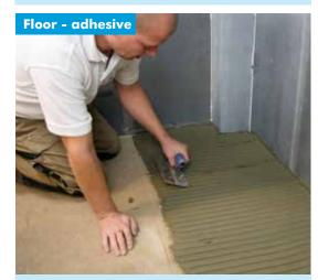
Use a floor trowel to comb the adhesive onto the floor.
