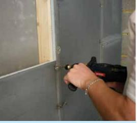
**2** Use a screw/Marmox washer every 300mm on each stud. When stud is at 600mm centres, use 20 rows of 5 fixings. At 300mm centres, use 3 rows of 5 fixings.
