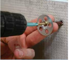
**2** Marmox Multiboards can be fixed to solid wall with screws and washers at every 300mm.
