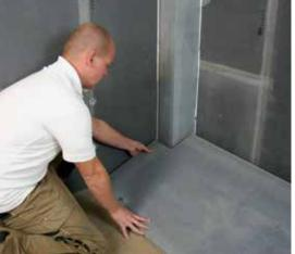
Lay the Marmox Multiboard down onto the adhesive and push firmly.
