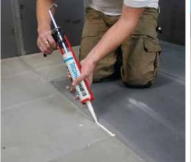
You can use Marmox Multibond for further waterproofing or in really wet areas use Marmox Self Adhesive Waterproof Tape.
