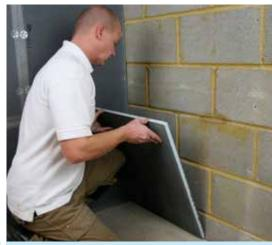
**2** Push firmly onto wall. Ideally stagger the joints.
