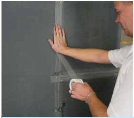
**3a - Tiling**. Be sure to tape all the joints with Marmox Reinforcing (scrim) Tape, except in wet areas where Marmox Self-Adhesive Waterproof tape should be used. The boards are now ready to be tiled.
