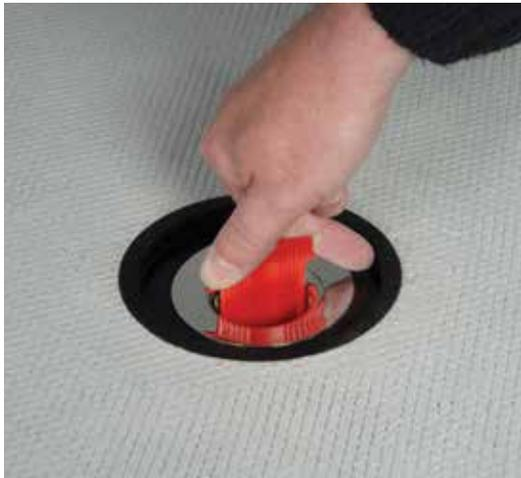
**7** Screw the flange ring through the Showerlay into the drain below. Hand-tighten using the red "key". No sealants should be used.
