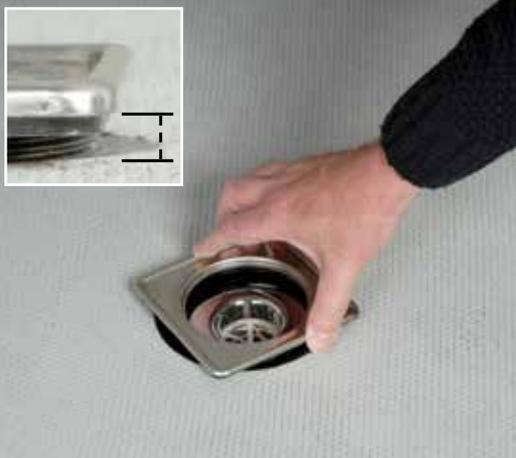
**10** Twist to align the height of the drain frame with the height of the tiles. For tiles thicker than 12mm additional drain frames may be stacked to reach the desired depth.
