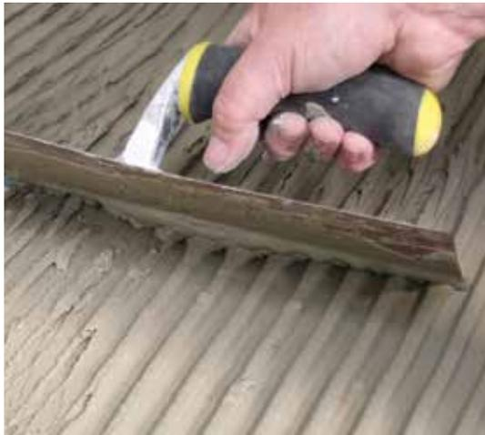
**6** Using a cement-based flexible tile adhesive, stick the Showerlay to the floor, checking again that it is level.
