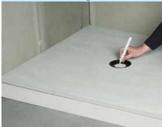
**A** The 100mm thick plinth will encase the drain and support the Showerlay.
