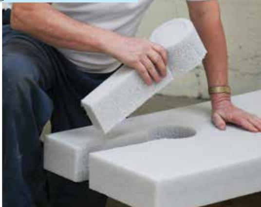
**B** Cut out a hole for the gully (diameter 130mm – 150mm) and a channel for the drain pipe.
