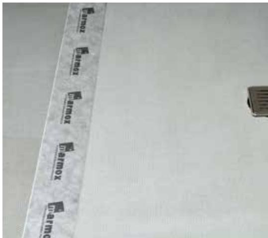
**9** Tape joints using Marmox Self-Adhesive Waterproof Tape.
