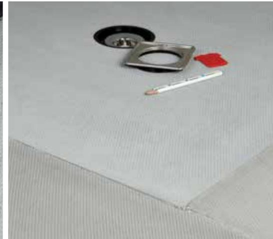
**8** If using a 20mm thick Showerlay, the rest of the floor can be raised to this height with Multiboard 20mm.
