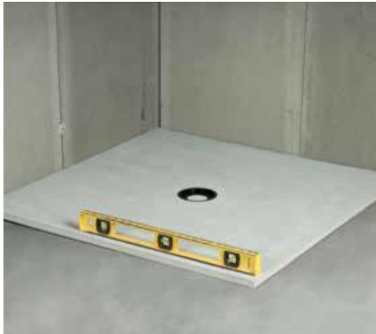
**5** Check that in position, the Showerlay is on a flat surface offering support – especially around the drain.
