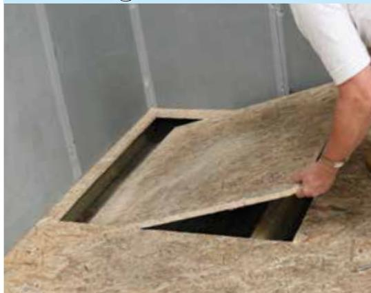
**A** Decide where the Showerlay is to go, draw around it and cut the floor section out using a jigsaw.
