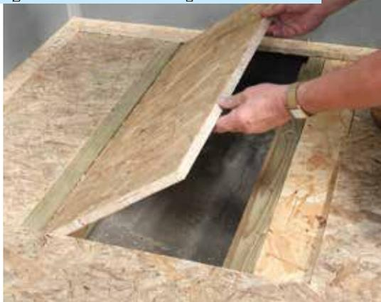
**B** Make support shelves with the cut up flooring and battens fixed to the side of the joists.
