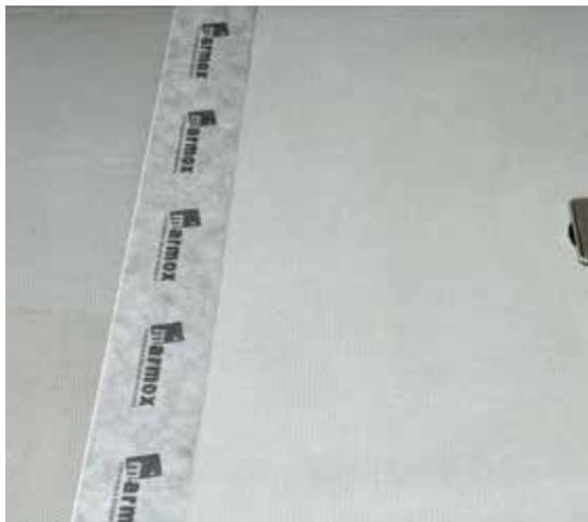
**9** Use Marmox Self-Adhesive Waterproof Tape over all the joints with the surrounding floor and walls. Waterproof corners may also be used.
