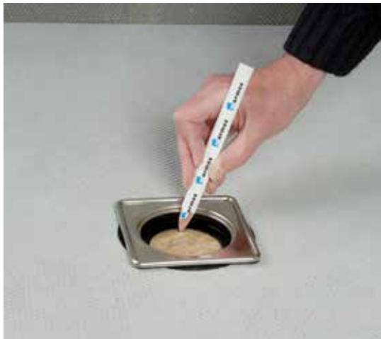
**1** Decide where the Showerlay is to go, then mark out the position of the drain hole.
