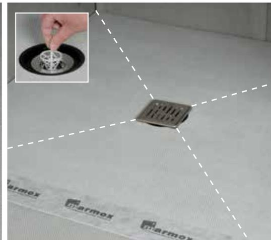
**12** There is no need to prime the unit, simply tile with cement-based tile adhesive. If tiles are greater than 10cm, they should be cut along the lines shown.
