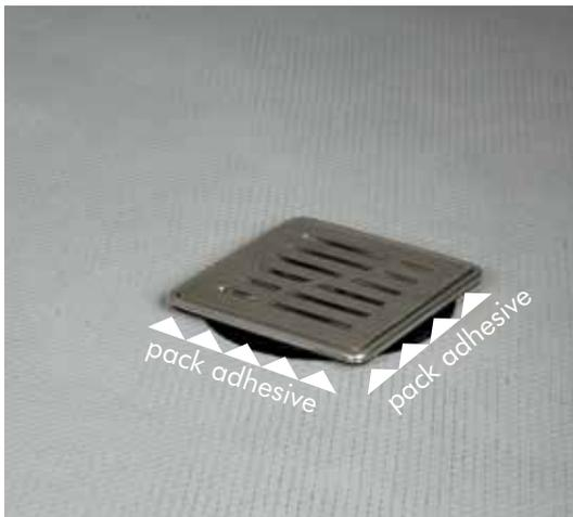
**11** Check that the height of grate in the silver frame will be level with the tiles when fixed with adhesive. To secure and stabilise the drain frame, pack some tile adhesive underneath.
