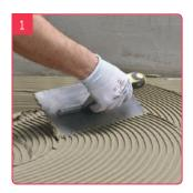
Spread tile adhesive Spread a flexible cement based tile adhesive over the floor
