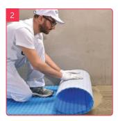
Lay the membrane Roll the membrane out over the whole floor and press into the adhesive
