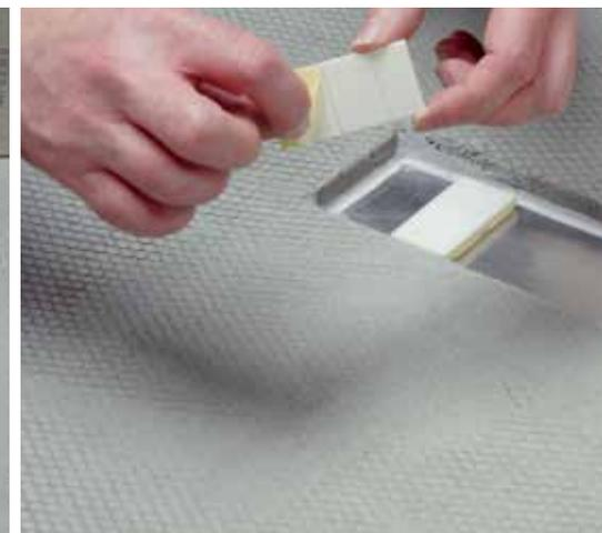
**8** If the height needs to be increased further, additional 2mm thick spacers can be stuck on top of the other spacers
