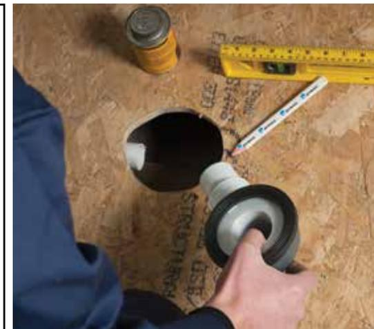
**4** Solvent weld the drain to the BS40mm pipe so it is positioned centrally in the hole.
