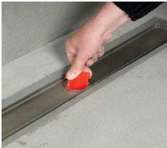
**9** Screw the flange ring through the Showerlay into the drain below. Hand-tighten using the red "key". No sealants should be used.
