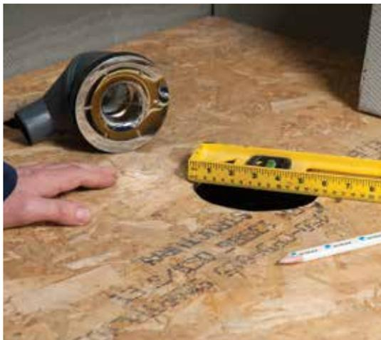
**2** Draw a larger circle around the hole with a diameter of between 130mm to 150mm and cut this out using a saw.
