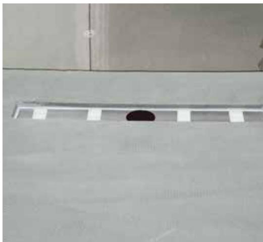
**7** Stick the four 4mm self-adhesive pads to the metal base of the Showerlay.
