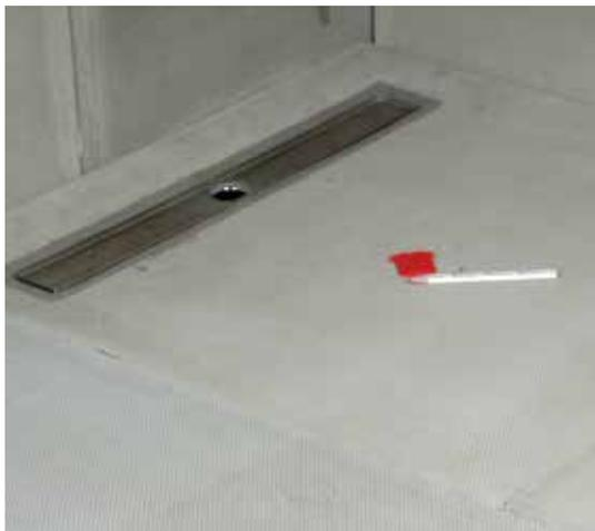
**10** Showerlay-Linear are 40mm thick. The rest of the floor can be raised to this height using Multiboard 40mm.
