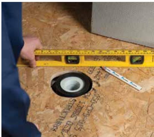
**5** Ensure that the floor is level and clean. Using a cement-based flexible tile adhesive, stick the Showerlay to the floor and position the drain tray into position.
