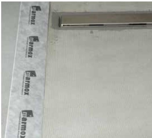
**11** Waterproof all the joints using waterproof tape and waterproof corners then fit the decorative grate, having first inserted the hair trap.
