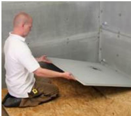
**1** Decide where the Showerlay is going to be positioned and make sure the area is clear and dirt free. Lay the Showerlay down into place.
