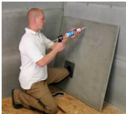
**7** Using Marmox Acrylic Sealant or alternatively a good quality cement based adhesive, stick the Showerlay to the floor.
