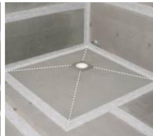
**16** If using tiles larger than 10cm on the Showerlay they should be cut along the lines shown above.
