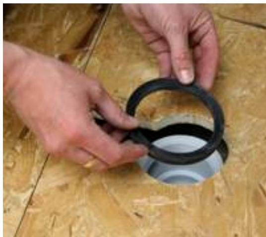
**5** Place the black rubber ring onto the top of the Dallmer drain.
