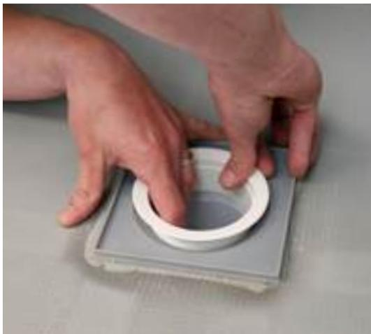
**9** Screw the plastic ring through the Showerlay into the Dallmer drain making sure the black rubber ring is in position.
